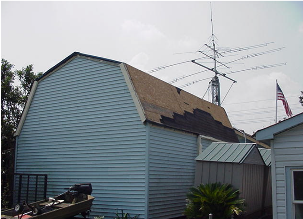
Holy Innocents also sustained severe damage to the roof of the Church and Rectory, and rain damage to the Church interior, vestmants and other items.
